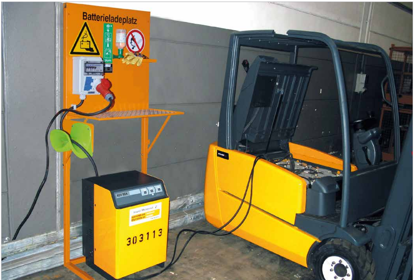
BL with CEEform socket 400 V charging the battery of an electric forklift truck
