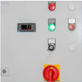
Switch cabinet with digital temperature display
