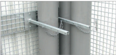
Fixture with safety chain
